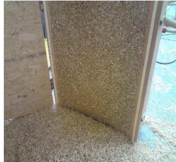
Thermal insulation material of wood chips and clay (instead of boron)
