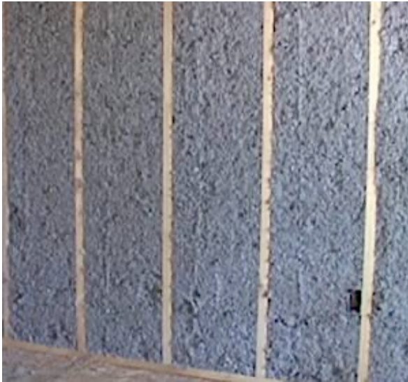
Cellulose insulation dampsprayed
